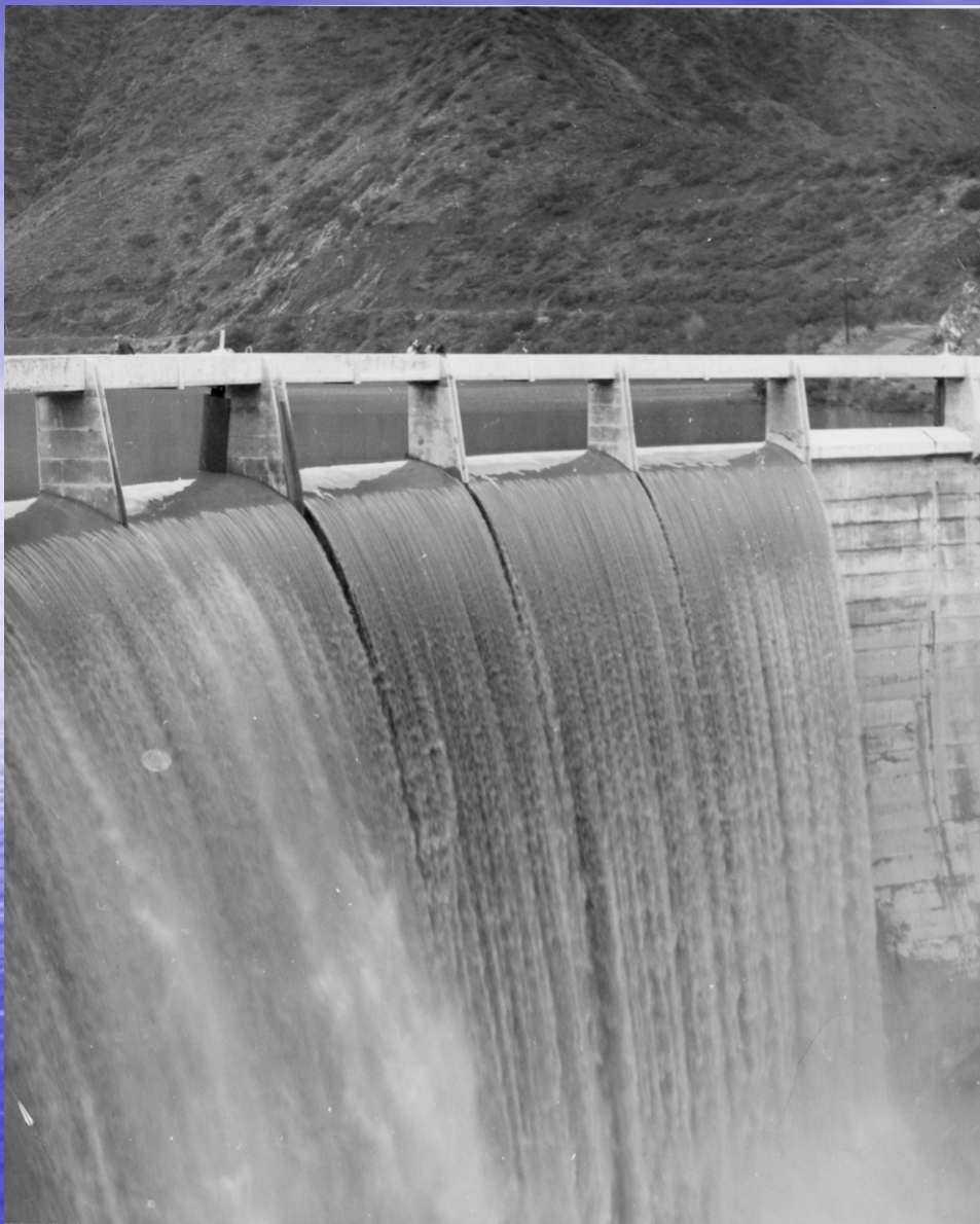
Initial spillage in 1952. Note people standing on 8-foot wide walkway for scale. The design capacity was 60,000 cfs
